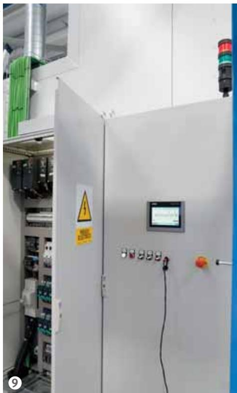
**Figure 9: The plant is equipped with the most sophisticated control systems of the parameters, the process conditions and the functioning of the entire line through a Siemens PLC.**
